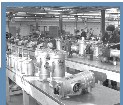
Brassmill Lane factory floor in the early 1970s
