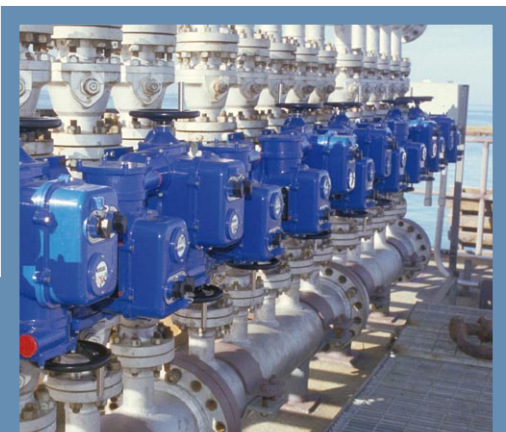
Some of the thousands of 'Q' Range actuators fitted to oil well head manifolds on Lake Maracaibo
