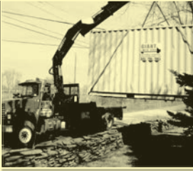
CRANE TRUCK DELIVERY
