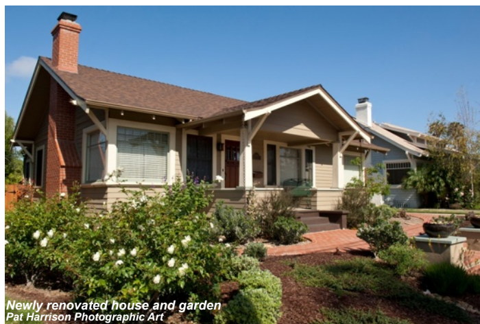
Renovation underway Pat Harrison Photographic Art
