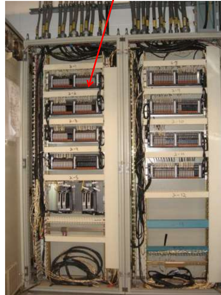
DeltaV CHARMs IO Panel post-upgrade 24 I/O Baseplate Migration Panels
