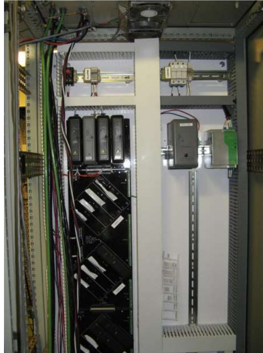
New Hardware pre-mounted on backplane
