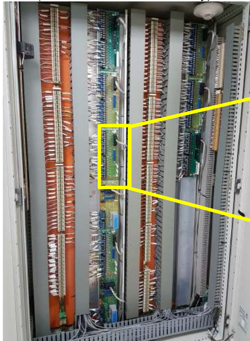
Typical Marshalling I/O FTA Cabinet (Field Termination Assembly)
