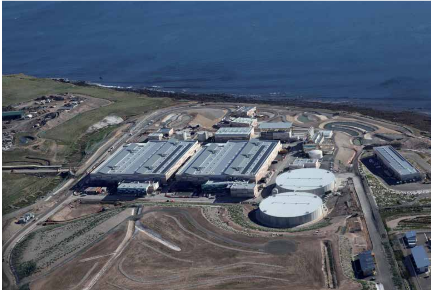
Port Stanvac desalination plant, Adelaide, Australia
