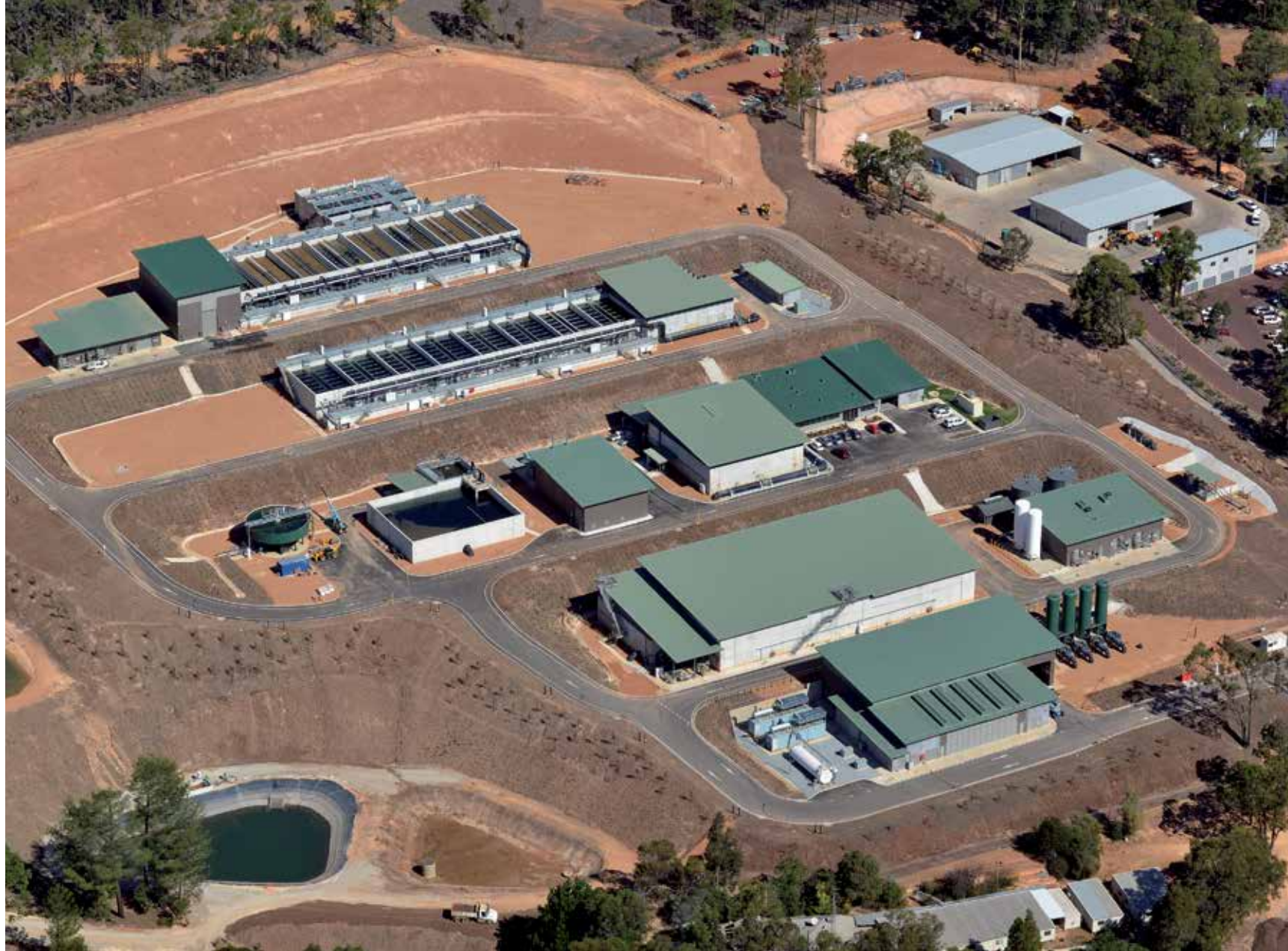
Mundaring DWTP, Perth, Australia
