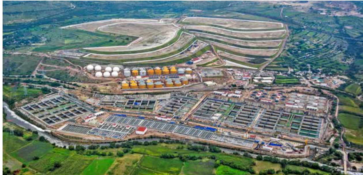
Atotonilco WWTP, Mexico
