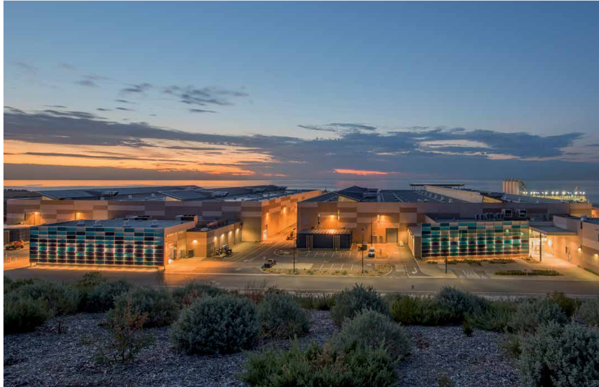
Adelaide Desalination Plant, Australia
