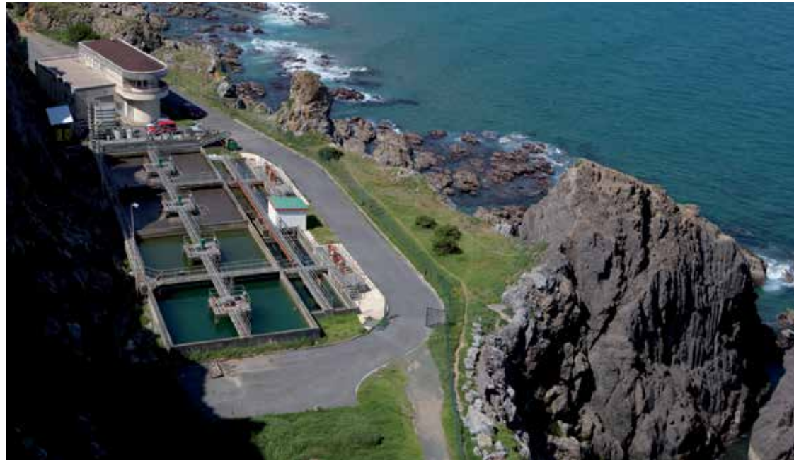
Bakio WWTP, Biscay, Spain
