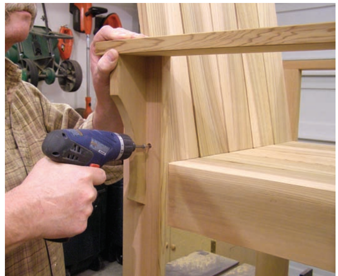
Drive a pair of 2" screws through each side of the leg sets to attach the backrest in place. The screws should anchor into the outside vertical slats, not the horizontal back braces.
