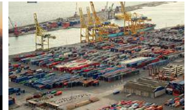
MATERIAL HANDLING PLANTS
