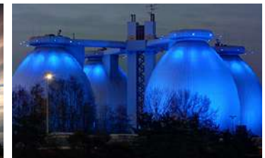
WATER TREATMENT PLANTS
