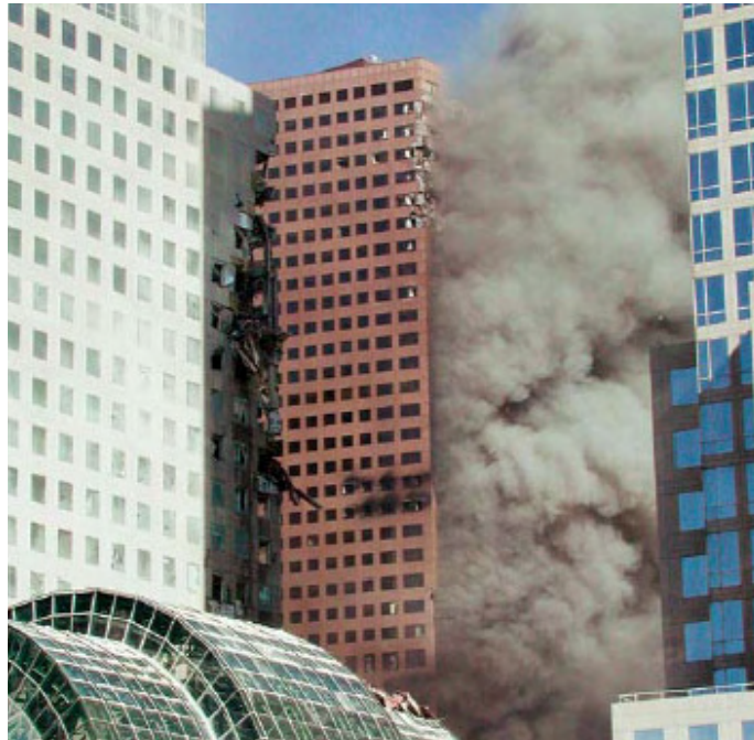
(b) WTC 7, South Facade/Corner
