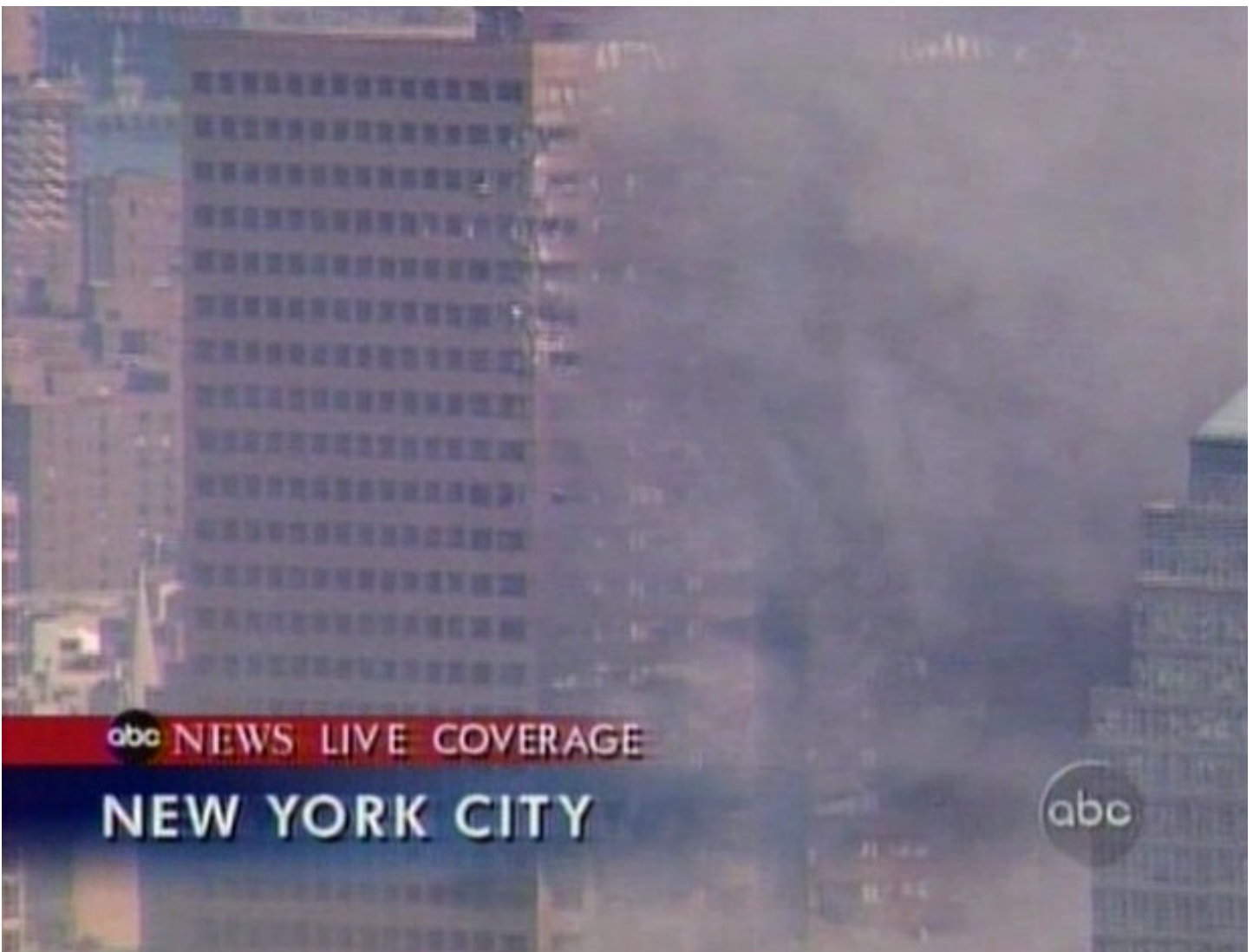
(c) WTC 7 , South Facade,
