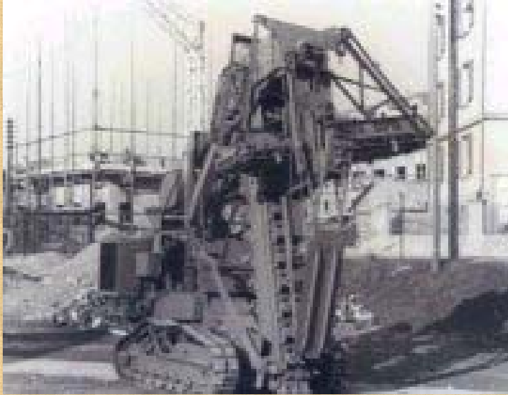
The first bucket trencher around 1943
