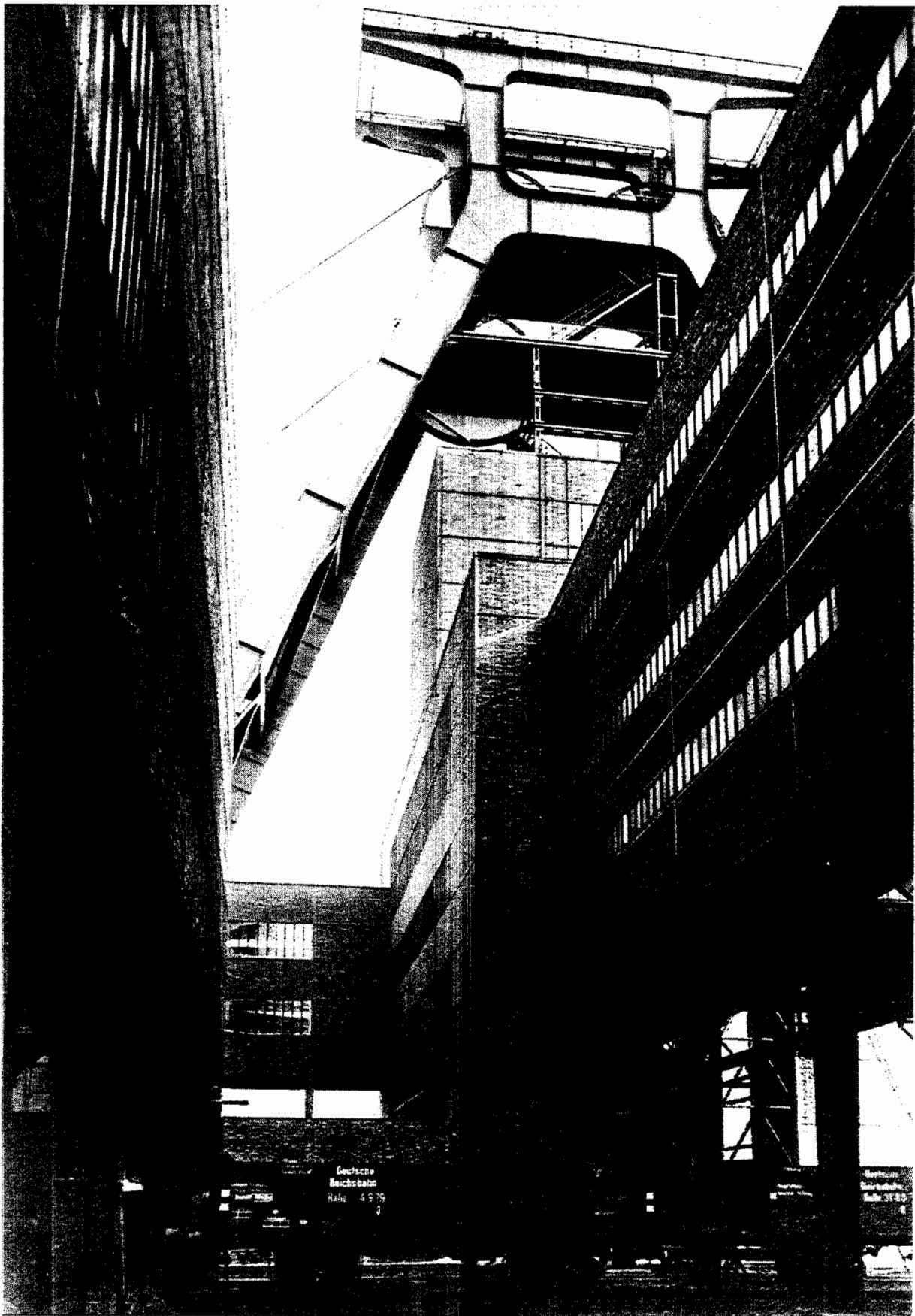
Essen, Zollverein Colliery Pithead 12, winding gear, shaft building (Photo: F. Schupp, Essen)
